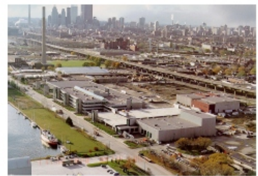
Structural Steel-Ontario Hydro Bldgs.
