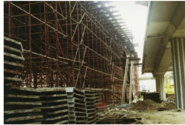
Scaffolding & Formwork-Hong Kong Bridge.
