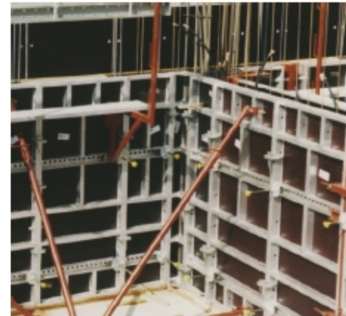
Aluminum Wall formwork-Japanese Hotel.
