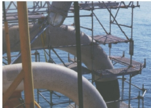
Access Scaffolding-Gulf of Mexico Oil Rigs .
