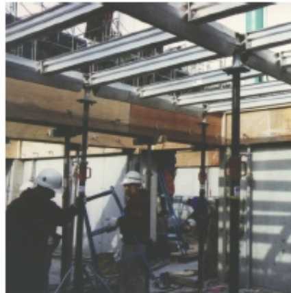
Slab formwork- Japanese Hotel.
